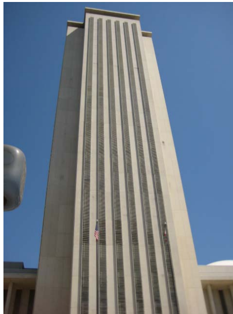
Florida's New Capitol Building, circa 1970
